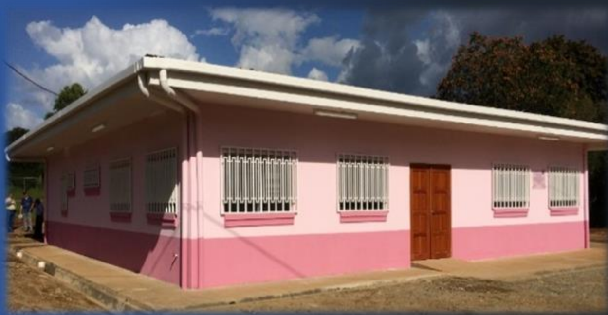
Maternal Homes in Las Quebradas Community, Siuna
