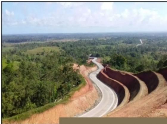
Improvements, extensions and construction of new roads
