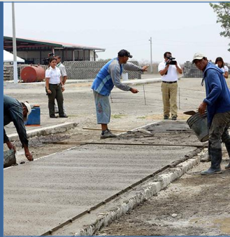
Construction and equipment of the Productive Complex and areas for attention and procedures in the Tipitapa complex
