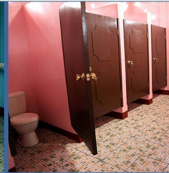
Rehabilitation of the hydrosanitary network in the Matagalpa, Tipitapa, Juigalpa, Granada and Estelí prisons.
